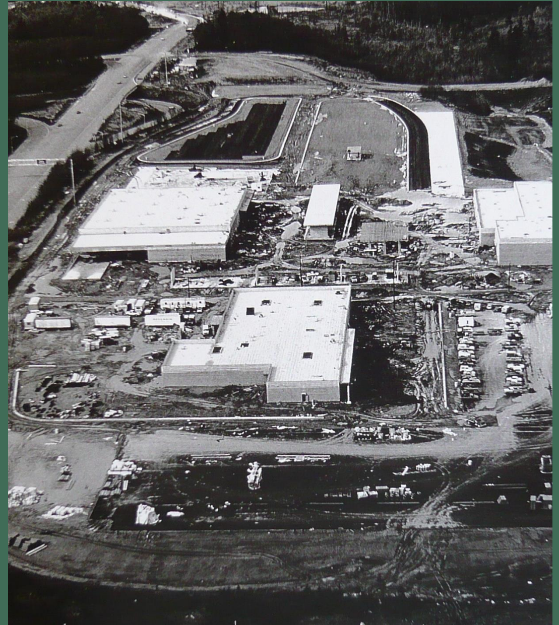
Operations Center Construction - 1980
