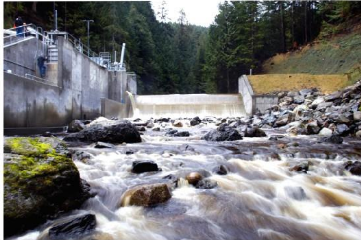
The PUD's Youngs Creek Hydroelectric Project generates enough electricity to power approximately 1,500 homes annually.
