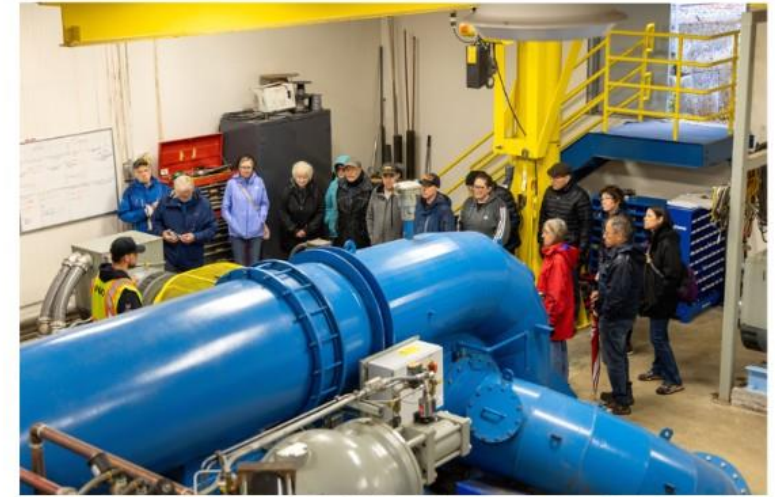
Community members gather in the generation house of the PUD's Woods Creek Sustainability Center, a run-of-river hydropower project.
