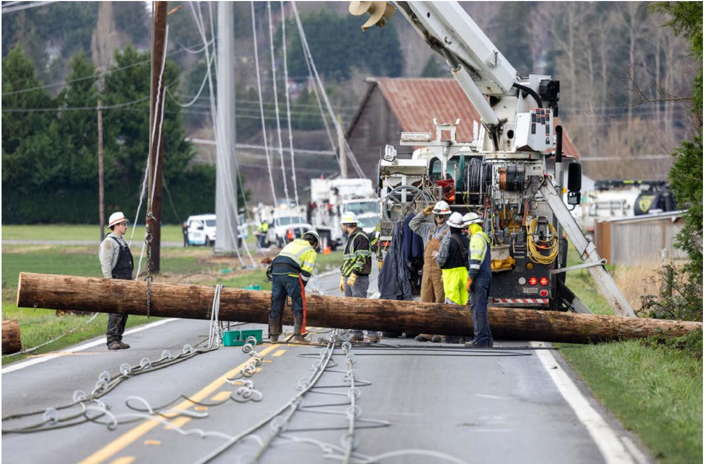
Crews work to restore power during an outage in December 2025.
