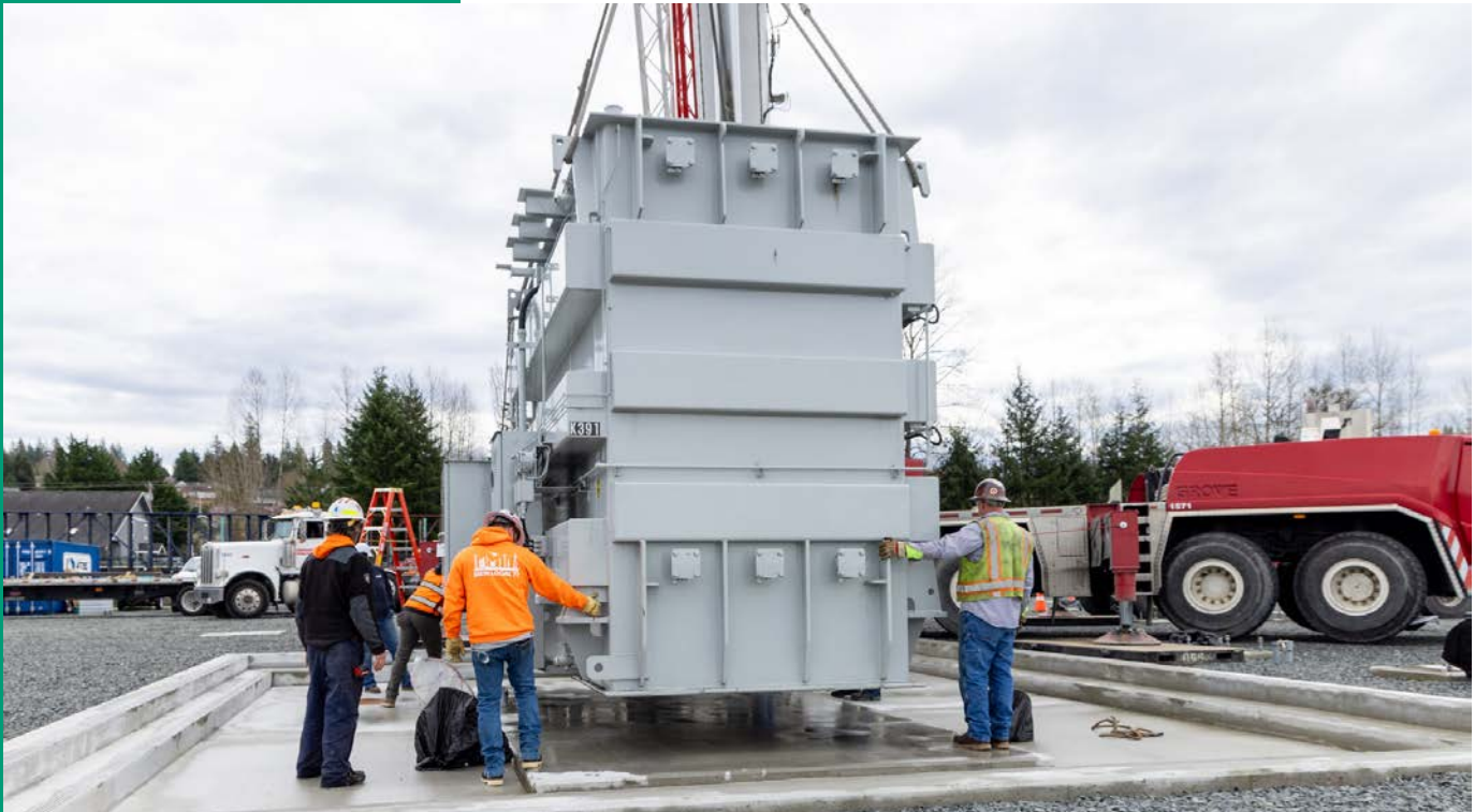
Installing a new transformer at the Crosswind Substation.
