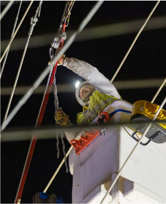
Moving lines in Sultan for a road project.
