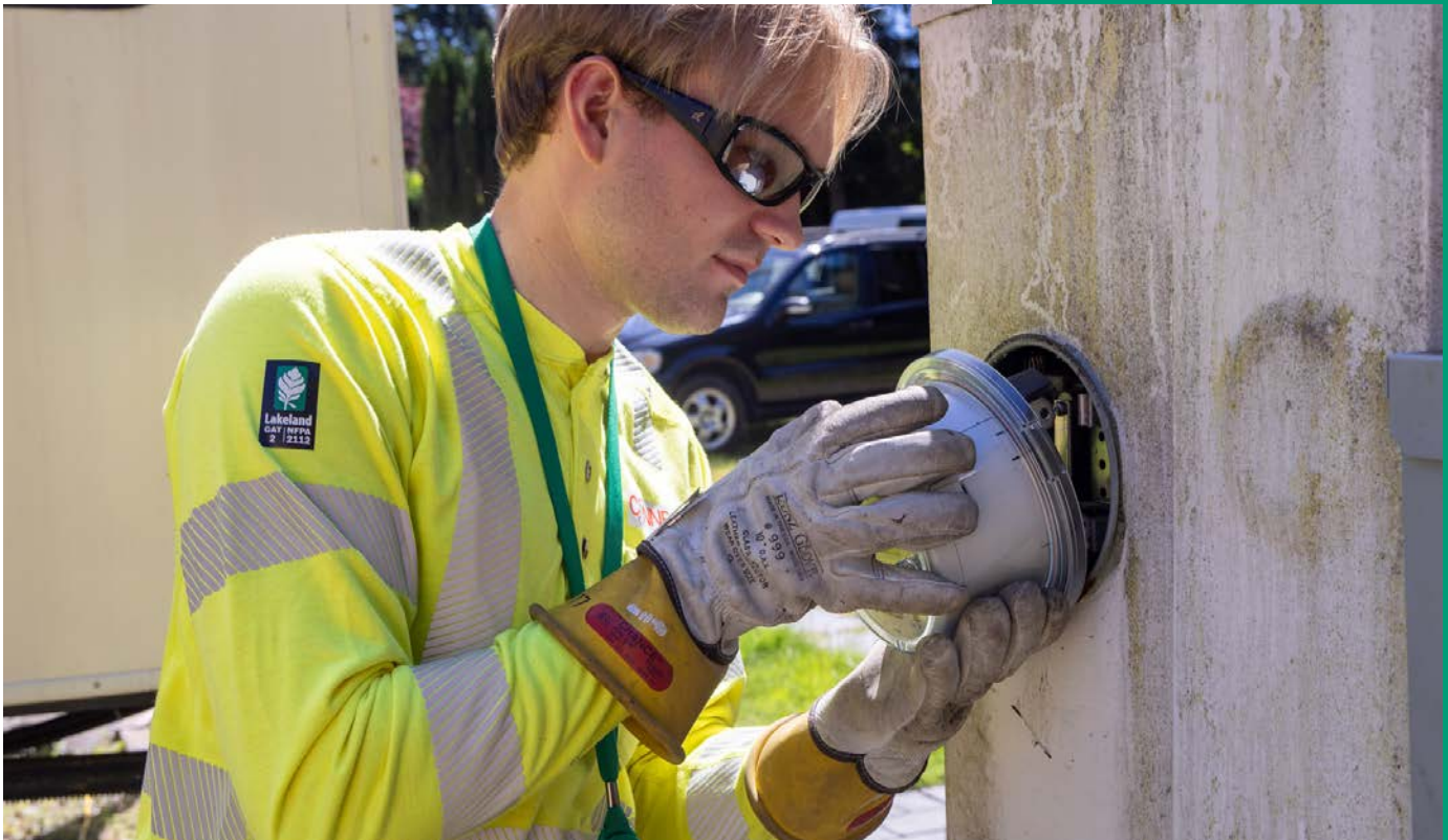
Installing a new meter as part of the Connect Up program.
