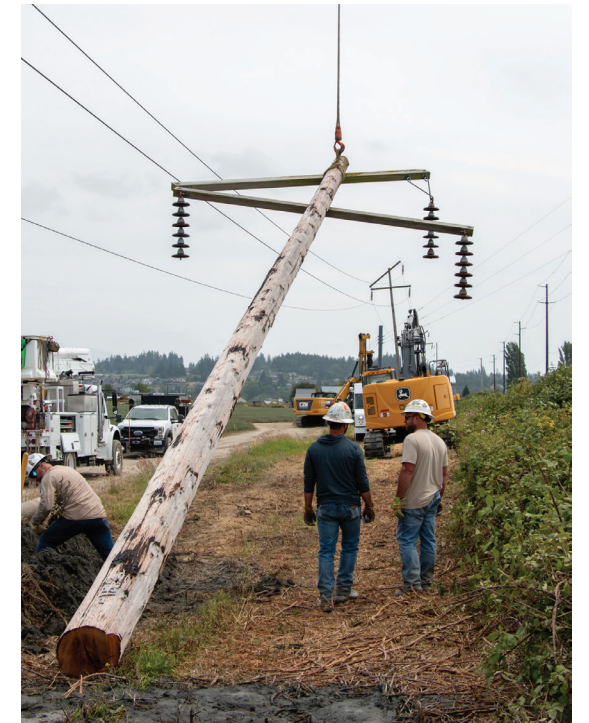
Pole replacement along the Stanwood-Camano line in late June 2025
