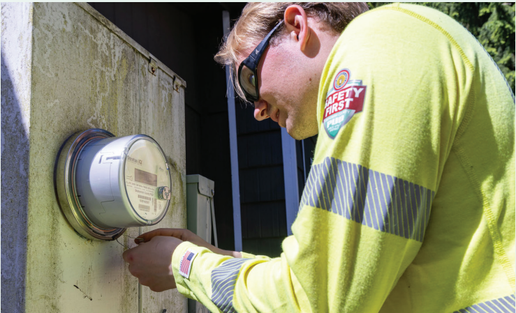
Connect Up meter installation near Echo Lake in May
