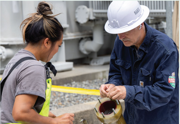
Maintenance work at the Jackson project in June
