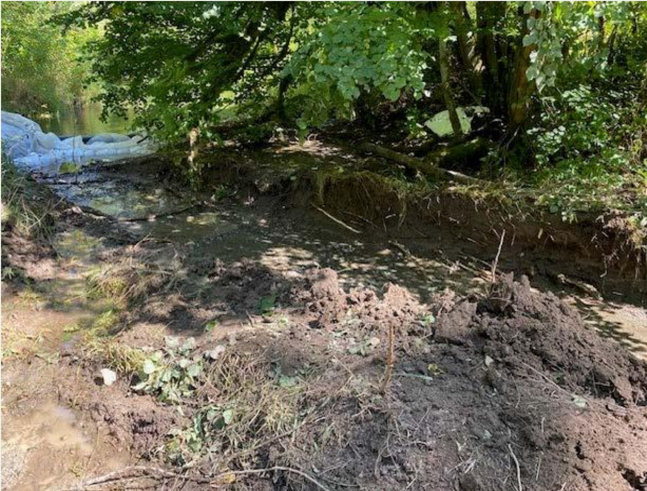
During Construction (August 2024)
