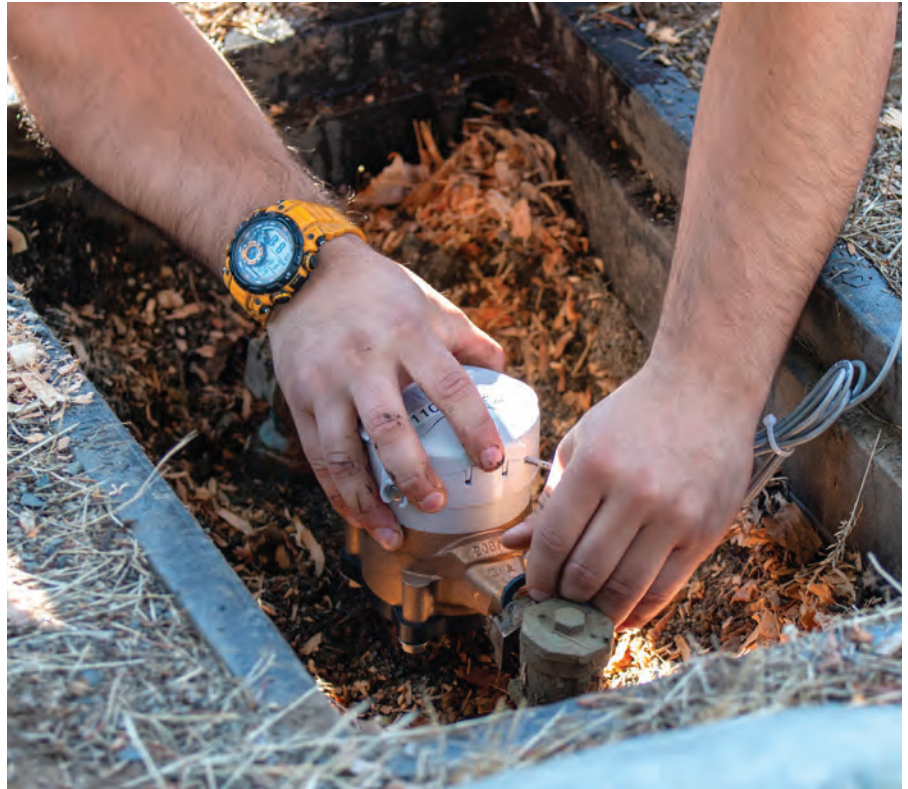
Above: PUD staff install a new advanced meter. Right: PUD staff testing the water.
