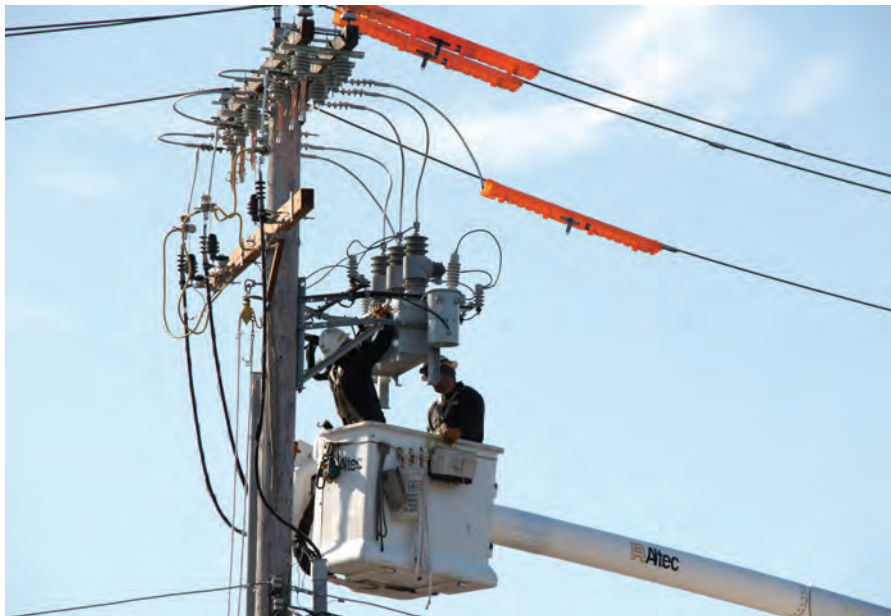
Above: PUD staff install a recloser for the SnoSMART program. Right: A Connect Up program van is ready to head out for installs.
