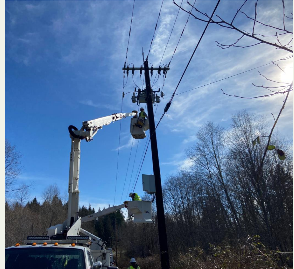
First DA Recloser commissioning in Arlington area as part of the project's proof-of-concept stage.
