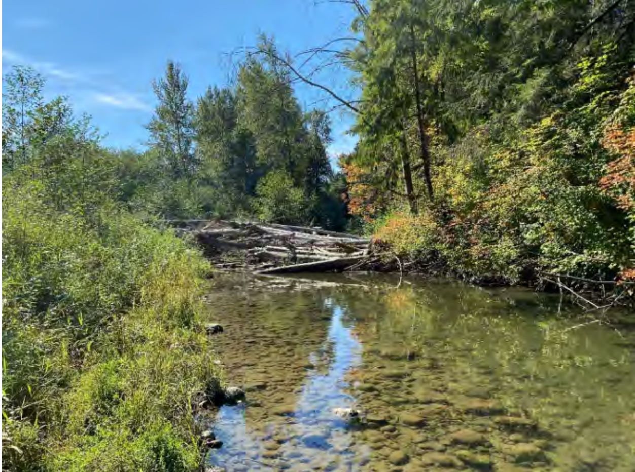
Figure 53. Racking of large woody debris on Engineered Log Jam 1 at the head of Side Channel 4 after Channel Forming event of 2020.
