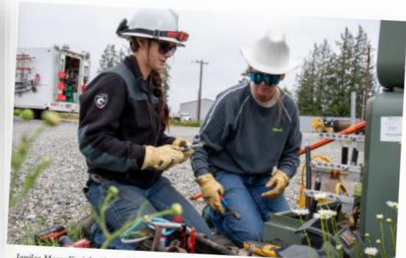
Jenilee Marzolf, right, demonstrates to Leigh Meyer-Beyer how to splice a secondary conductor at SnoPUD's Arlington Training Yard.
