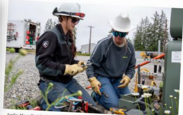
Jenilee Marzolf, right, demonstrates to Leigh Meyer-Beyer how to splice a secondary conductor at SnoPUD's Arlington Training Yard.
