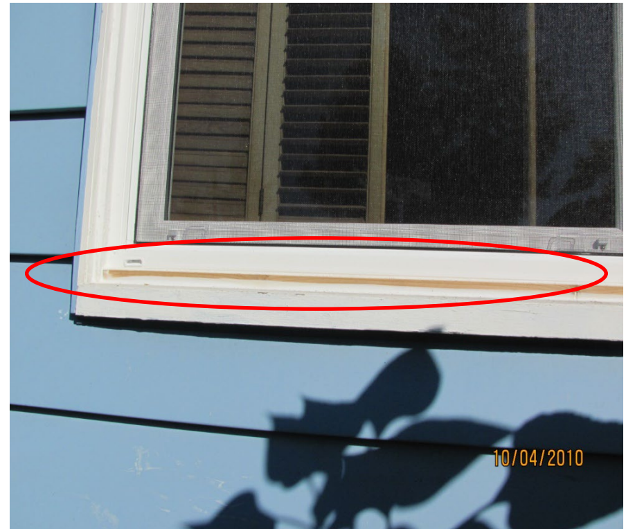
Wood Stopped Install (106.622)
