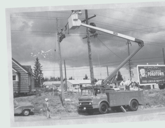
Above, a PUD crew installs a streetlight in the 1960s. Right, crews work on a Connect Up base station.
