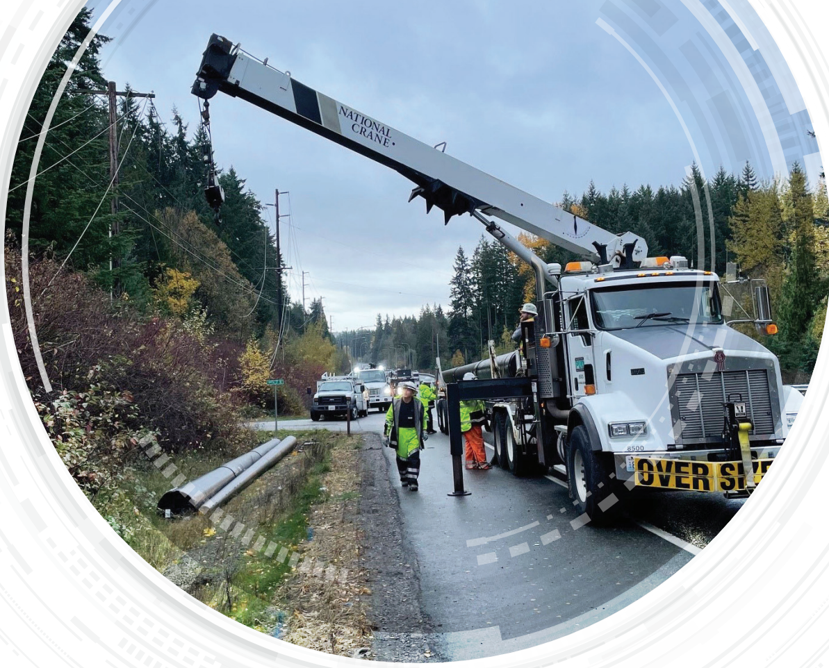
Crews repair storm damage along Highway 9.
