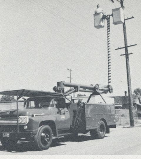
Used for line work and the tree trimming that was (and is!) vital to reliability, this bucket truck had a maximum reach of 48 feet. Workers operated the hydraulic lift with hand controls from the bucket. When used in tree trimming, this truck often rolled with a chipper and dump truck.
