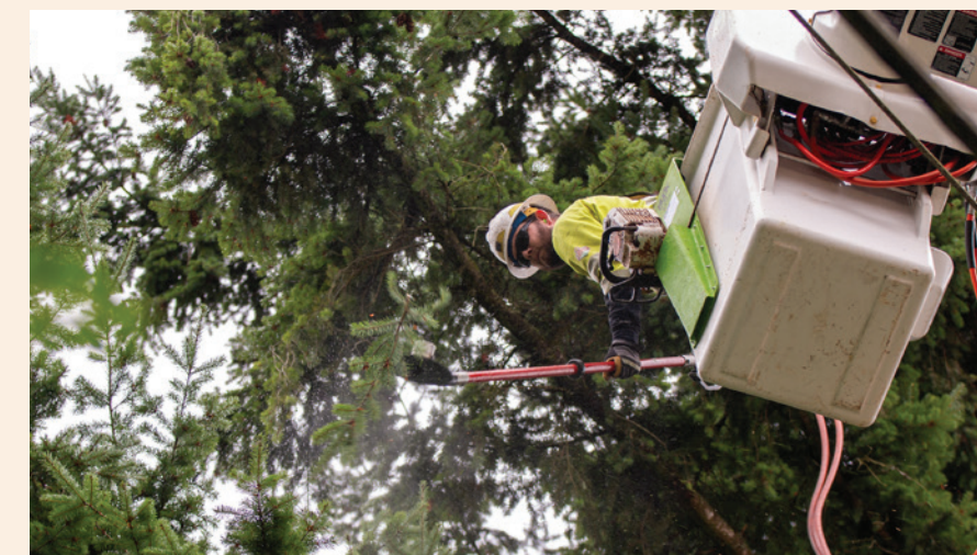
July > A PUD Tree Trimmer works in Lynnwood to clear branches well away from power lines.
