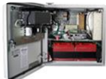
AMI Communications Network Deployment
