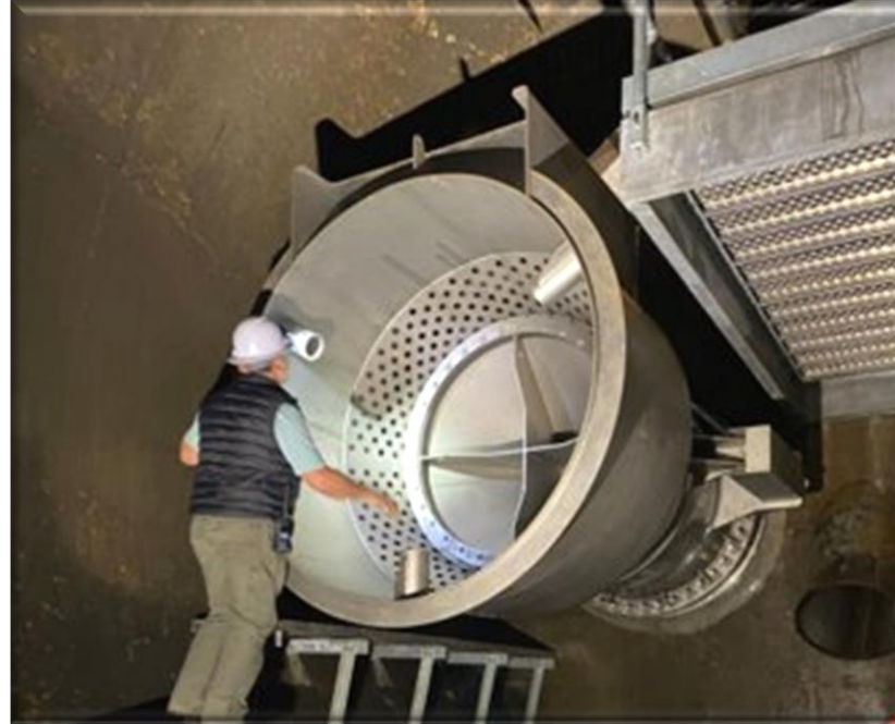
New 48-in valve installed and being inspected prior to commissioning
