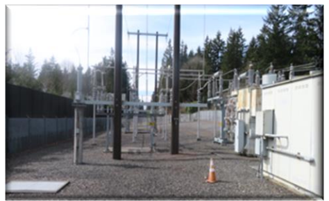
Brier Transformer & Switchgear Replacement
