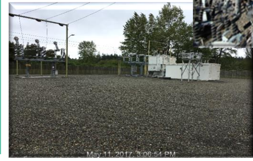
Camano Substation Rebuild
