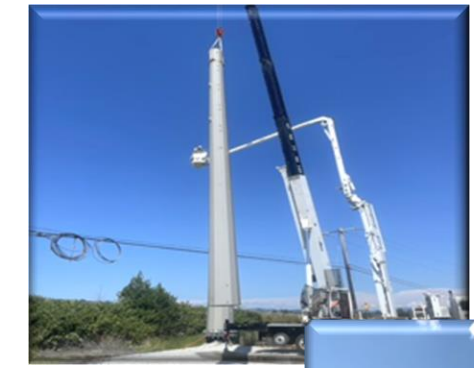
Stanwood to Camano 115KV Line Rebuild
