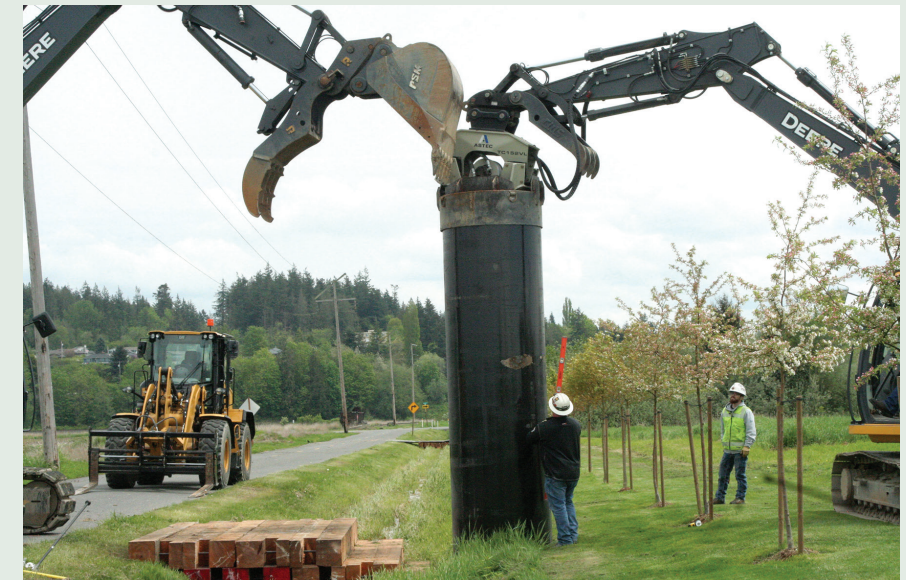
Work on the new Camano transmission line in May.
