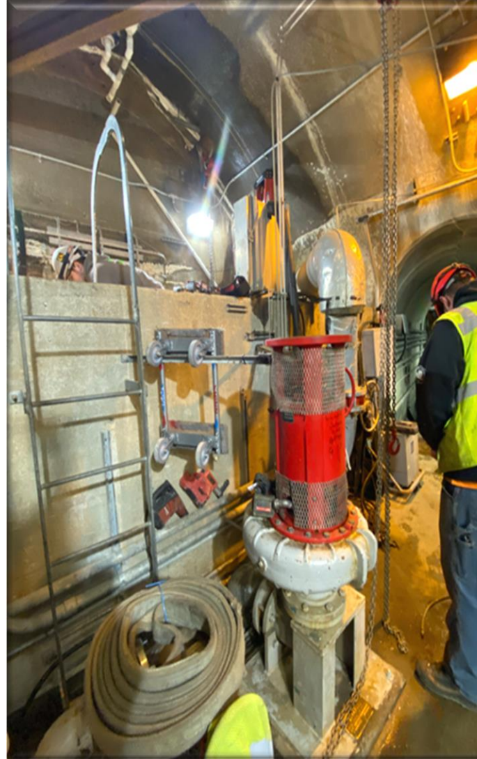
Decommissioning of the 60kw turbine/generator 230/243
