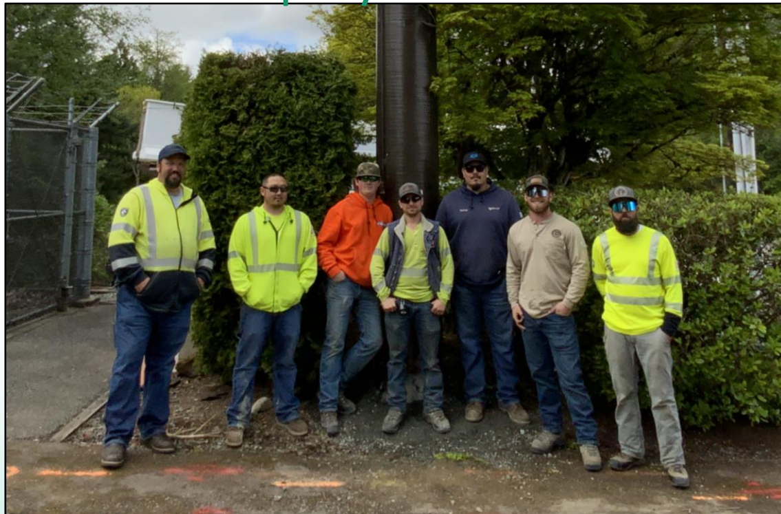
AMI Site 67 Installation, Hilton Lake Substation, May 9, 2023
