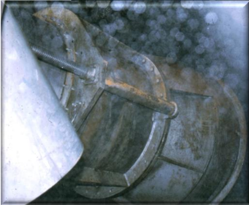
Replacement of end-of-life cone valves at the Jackson Hydroelectric project
