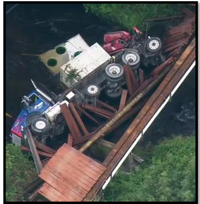
A private bridge at Woods Creek in Monroe that failed in September 2019
