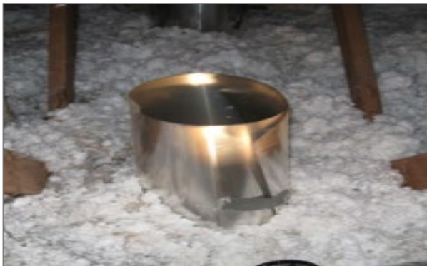
Recess light lashing and baffles
