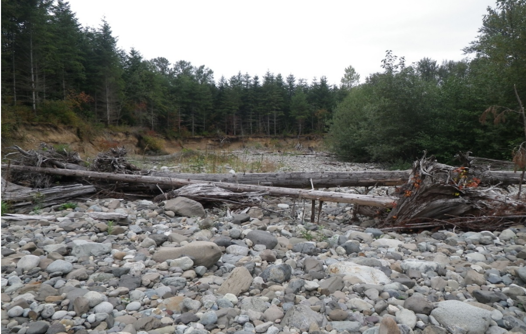
Photo C-33: Youngs Creek, main channel in dewatered state, downstream of Powerhouse near RM 2.1
