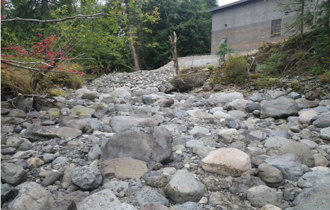
Photo C-8: Youngs Creek, dry channel immediately upstream of Powerhouse at RM 2.4 and location of dead trout presented in Photos C-1 through C-7
