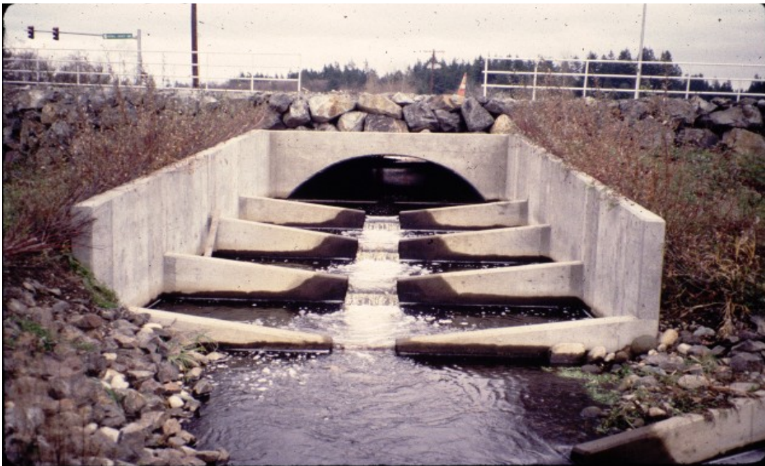
Figure 4-3. Example Photographs of Pool-and-Chute Fishways.
