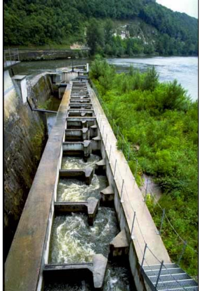
Figure 4-1. Example Photograph of a Vertical Slot Fishway.
