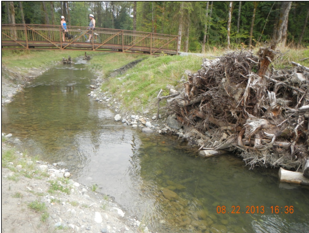
Figure 4-1. Redundant inlet to SC 1, looking downstream with Engineered Log Jam (ELJ) 4 on the right, mainstem discharge of 581 cfs.
