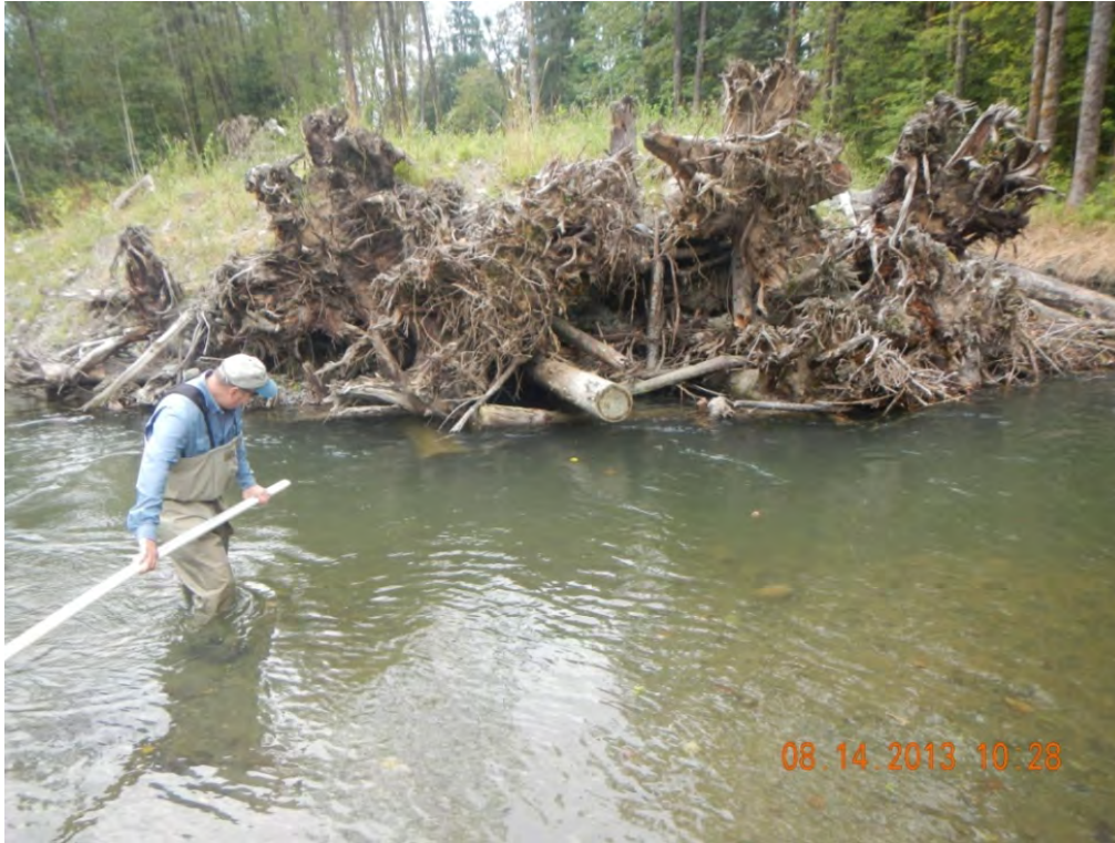
Side Channel 4: Engineered Log Jam 1.
