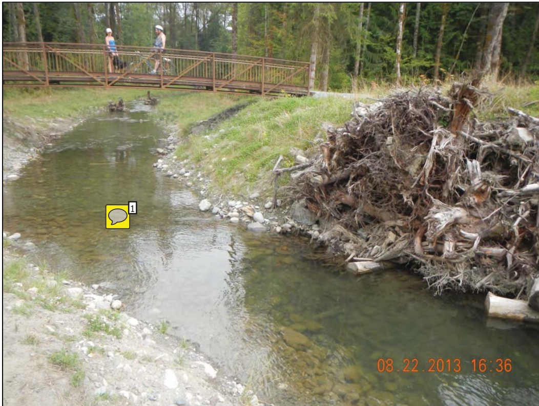
Figure 4-1. Redundant inlet to SC 1, looking downstream with Engineered Log Jam (ELJ) 4 on the right.
