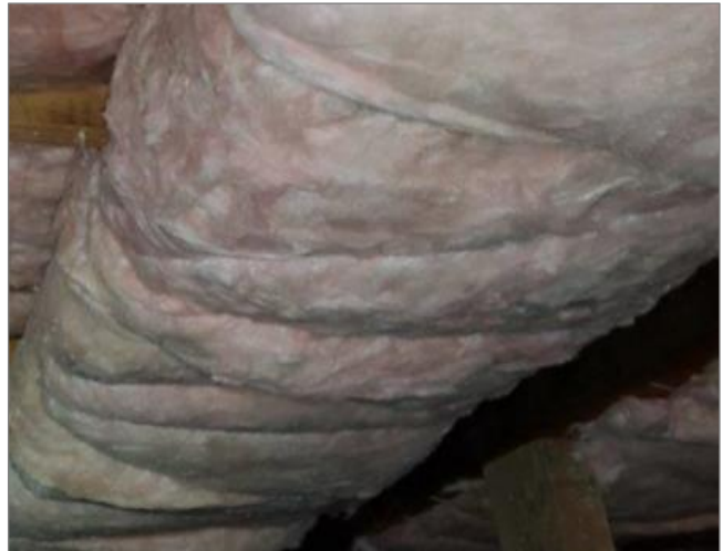
Two or three locations of insulated ducts wrapped with twine.
