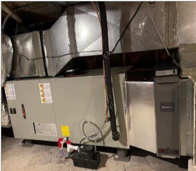
Installed Air Handler
