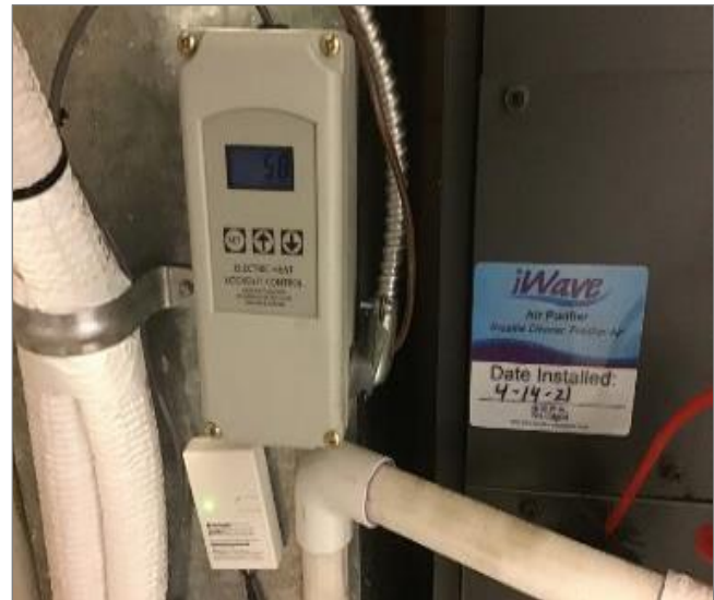
[If Mitsubishi] Auxiliary Lockout Controller located on air handler
