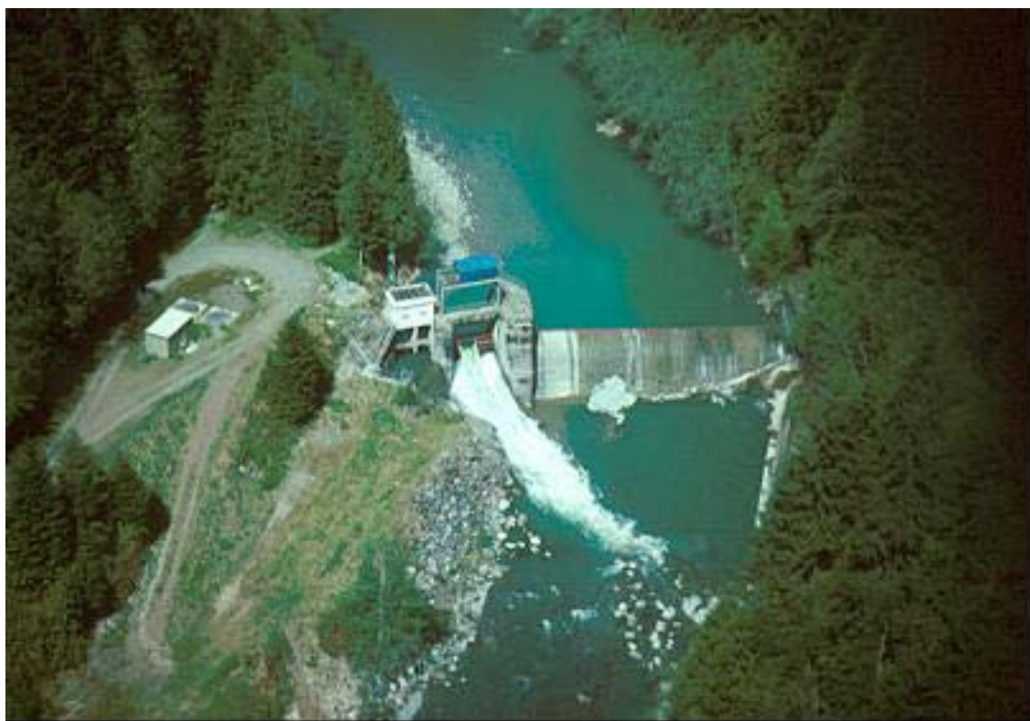
Figure 5 The Sultan River diversion dam at RM 9.7
