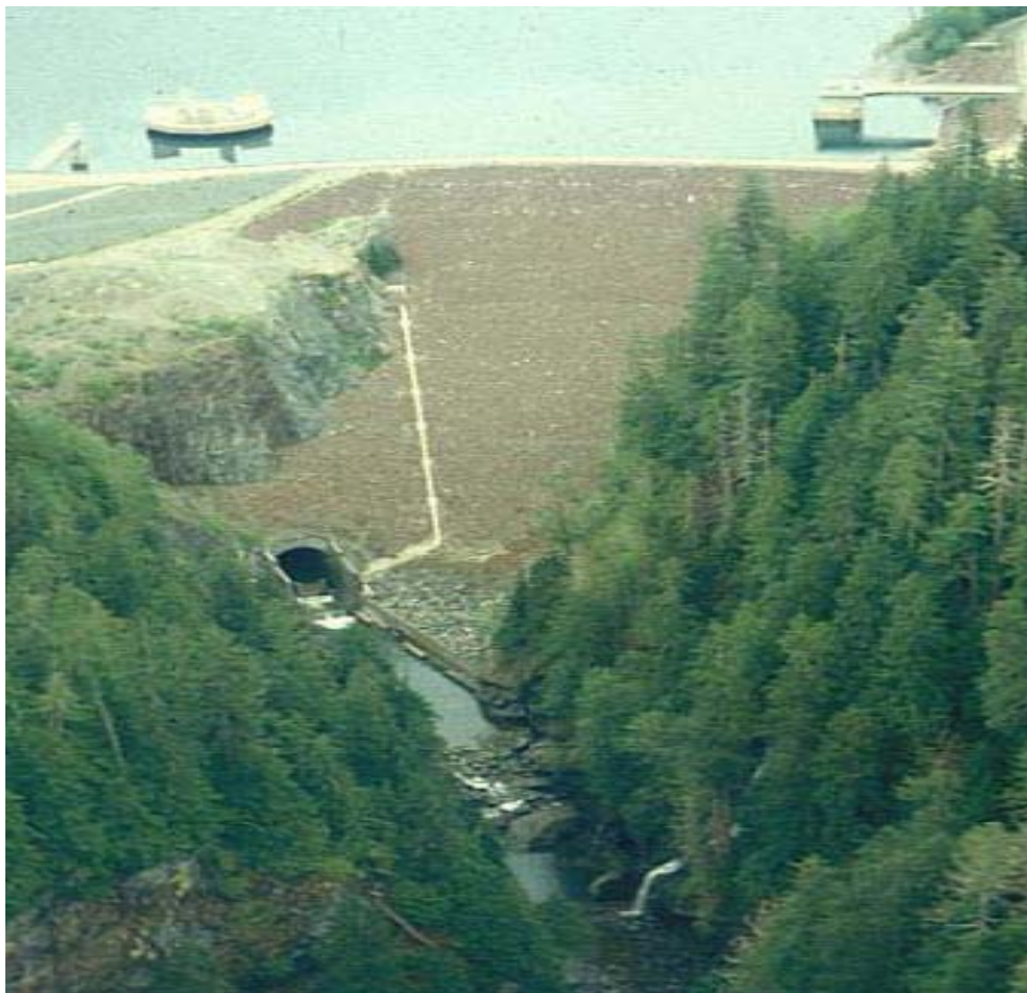
Figure 2 Culmback Dam and the morning glory spillway.
