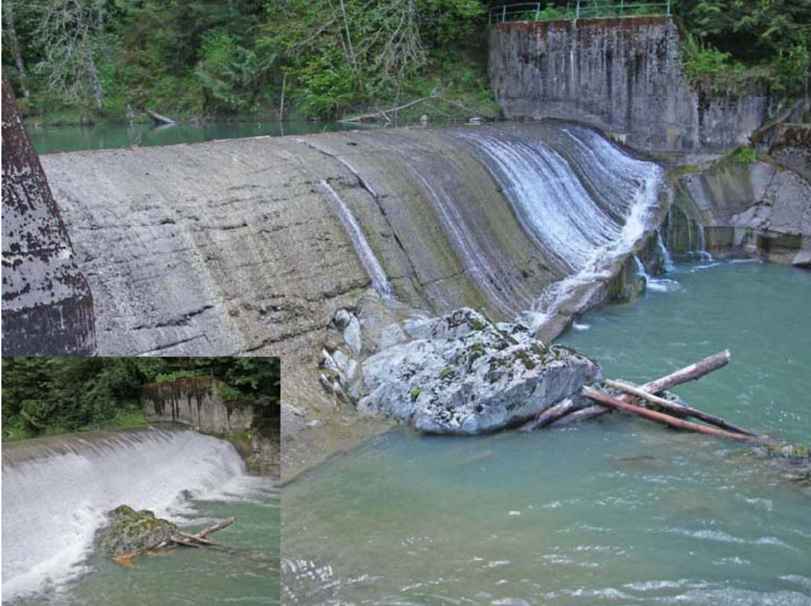
Figure E.6.3-26 The City of Everett's Diversion Dam located at RM 9.7 of the Sultan River.
