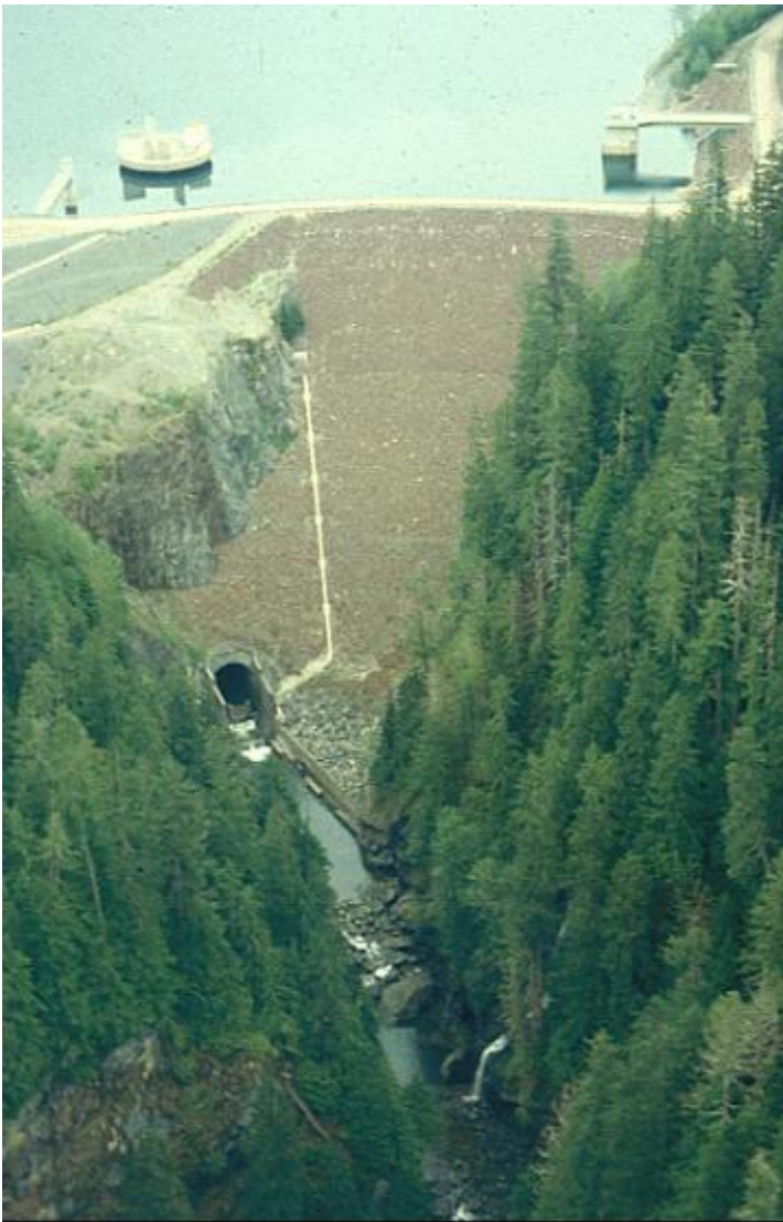
Figure A.2-2 Culmback Dam and the morning glory spillway.
