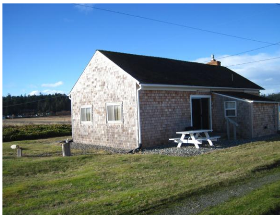
South and East elevations 2012
