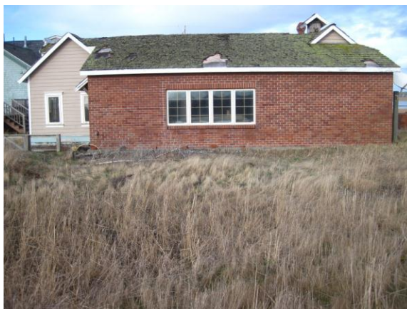
South elevation of garage 2012
