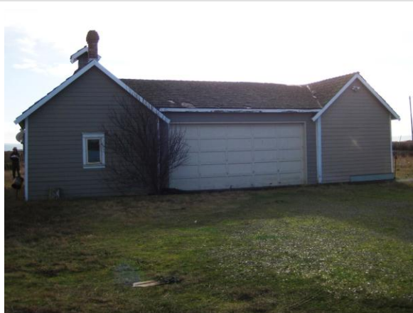
North elevation of garage 2012
