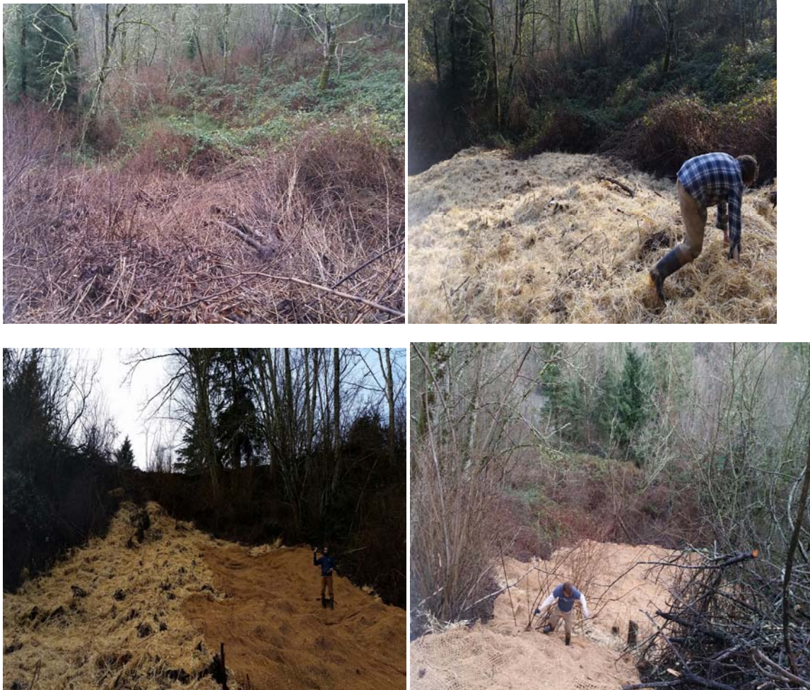
Figure 5: (Top left) Initial work area with knotweed can sticking up. (Top Right) Laying down straw after the site had been seeded. (Bottom Left) Starting to lay coir fabric on the slope, shingling each section. (Bottom Right) Complete coverage of the work area.
