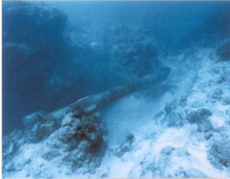
Figure 7. Drilling Head Exit.
