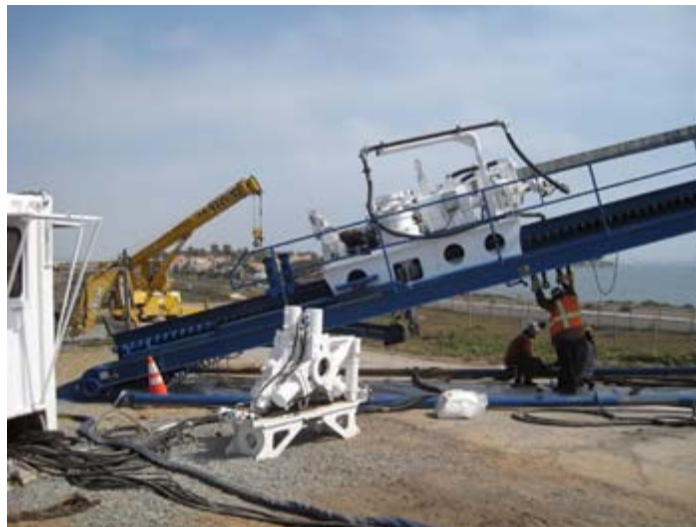
Figure 4. HDD Rig, View Two.
