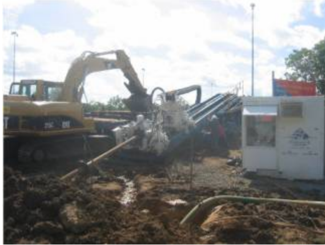
Figure 3. Typical HDD Set-Up.
